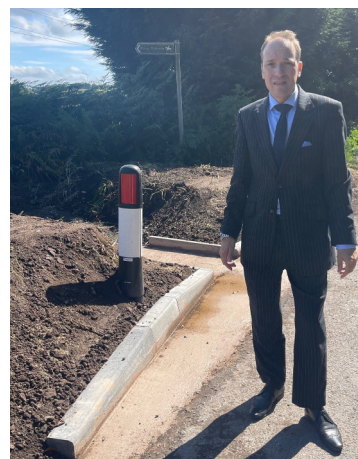
Safety verge markers and kerbing installed for Deansford Lane
